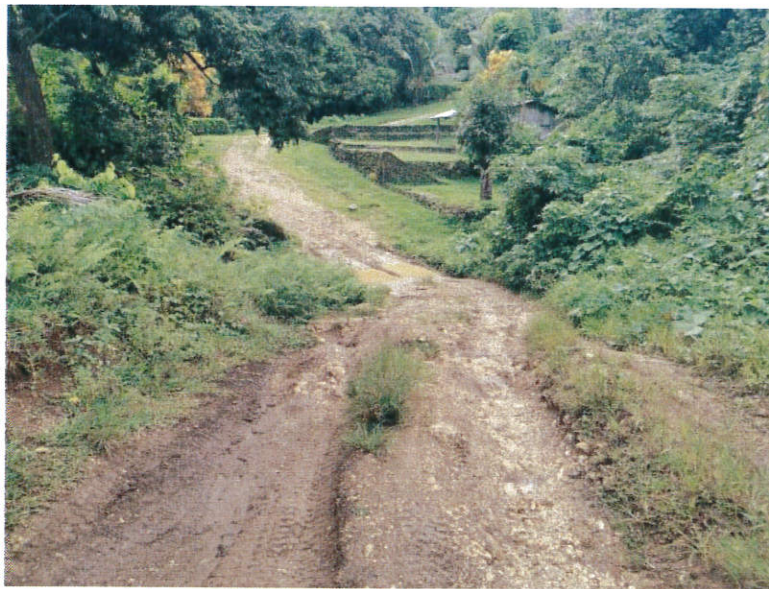
Figure 5. Road crossing a creek that normally floods during heavy rainfall. Conductor needs to be aerial. Typical soil composition (partially rocky) can be observed in this picture
